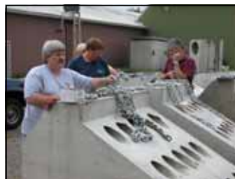
MAST members secure the mooring buoy chains to concrete blocks
