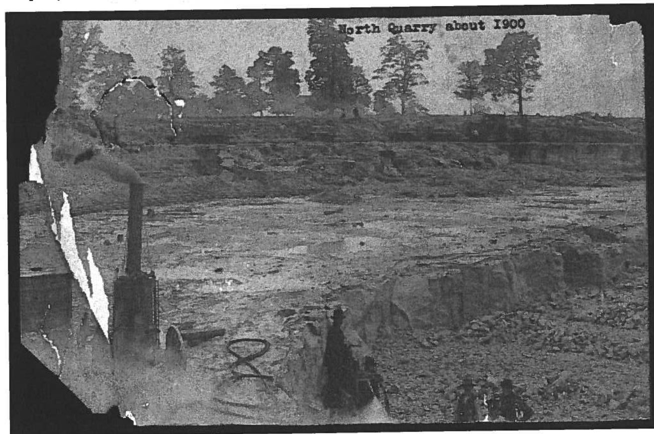
Figure 11. Kelley Island Lime & Transport Company's North Bay quarry, circa 1900 showing use of steam drill to bore blasting holes (Capt. Frank E. Hamilton Albums, Charles E. Frohman Collection, Rutherford B. Hayes Presidential Center at Fremont, Ohio). Note Shay engine and cars (upper right) transporting quarry stone.
