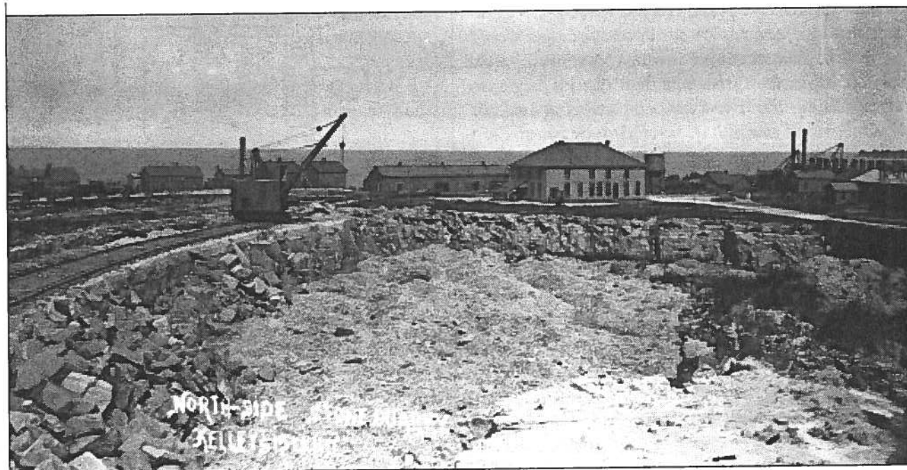
Figure 18. Kelley Island Lime & Transport Company's office building and company store at North Bay quarry, circa 1903 (Capt. Frank E. Hamilton Albums, Charles E. Frohman Collection, Rutherford B. Hayes Presidential Center at Fremont, Ohio). Note steam crane (whirly) on track at quarry's edge and crushed stone on quarry floor.
