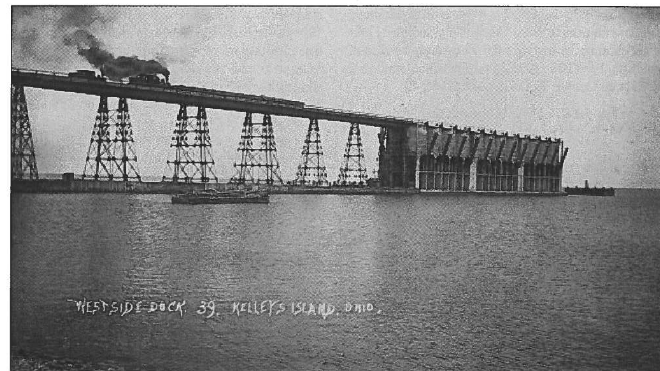
Figure 23. Kelley Island Lime & Transport Company's West Bay dock, circa 1925 (Capt. Frank E. Hamilton Albums, Charles E. Frohman Collection, Rutherford B. Hayes Presidential Center at Fremont, Ohio). Note Shay steam locomotives pushing narrow gauge dumping cars, loaded with crushed limestone, via a 600-foot-long overhead trestle to storage bins at the end of the dock. From the bins stone was loaded directly by gravity into bulk freighters.
