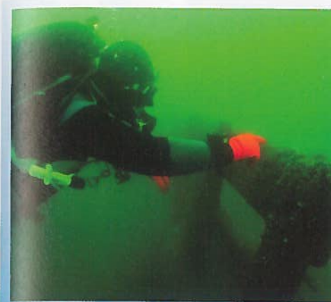
Intact port railing. Photo by David VanZandt, CLUE
