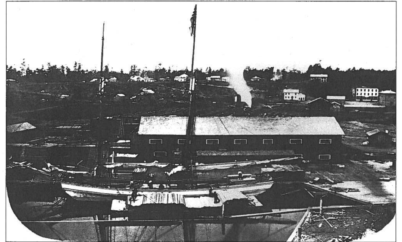
Scow schooner MILTON at Montague, Michigan (courtesy of Smithsonian Institution). Built at Milwaukee, Wisconsin in 1867, 102 x 24 x 6.8 feet. See modeler's plan of MILTON on page 26.
