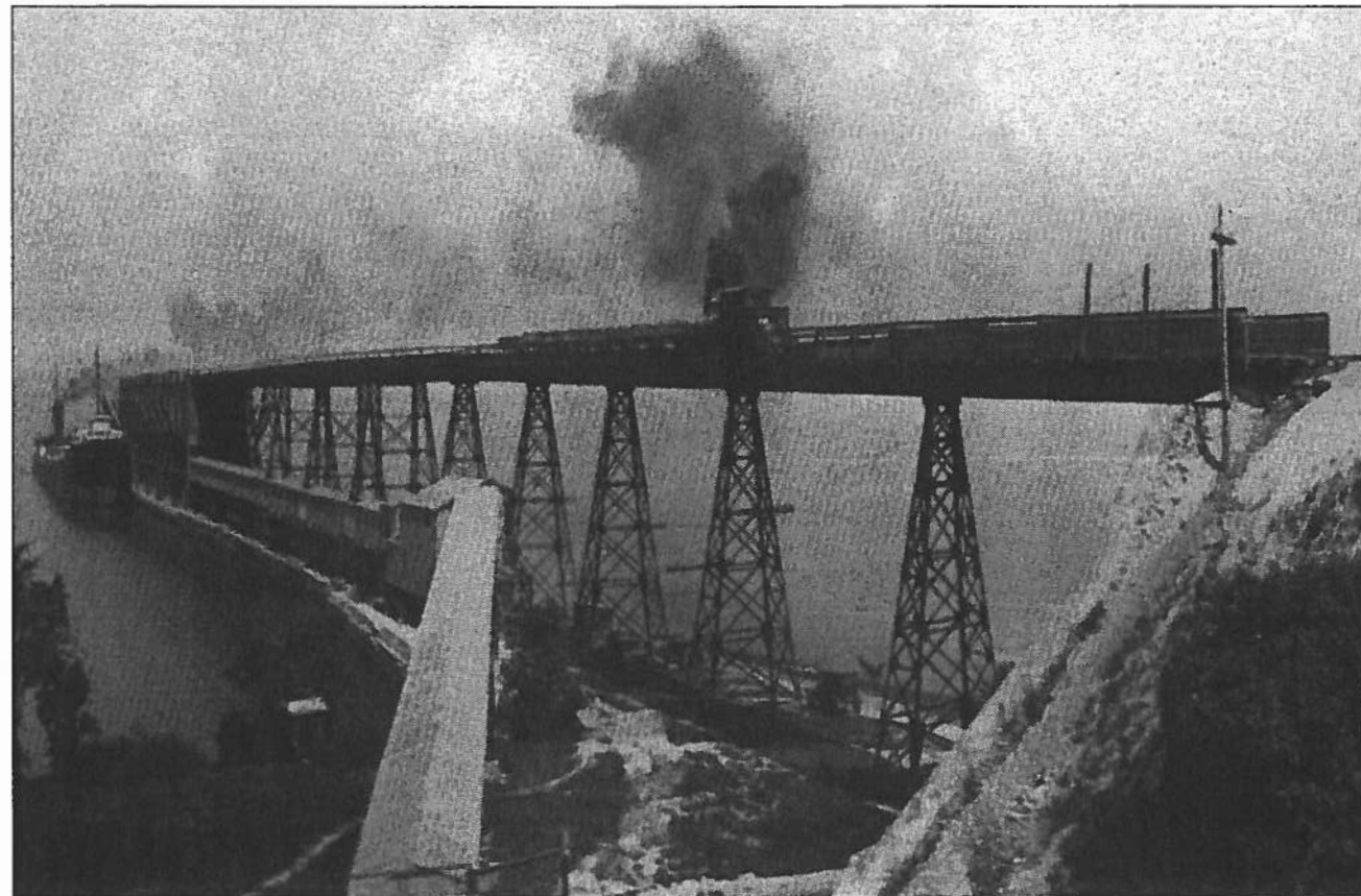
Kelley Island Lime & Transport Company's West Dock, circa 1925 (Capt. Frank E. Hamilton Albums, Charles E. Frohman Collection, Rutherford B. Hayes Presidential Center at Fremont, Ohio). Note Shay steam locomotives pushing narrow gauge dumping cars, loaded with crushed limestone via 600-foot long overhead trestle to storage bins at the end of the dock; from the bins stone was loaded by gravity directly into bulk freighters.
